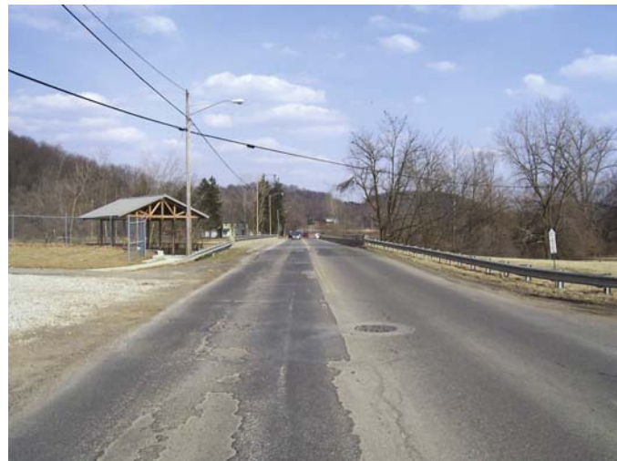
Waterworks Road at the bridge over the North Fork of the Licking River looking east
